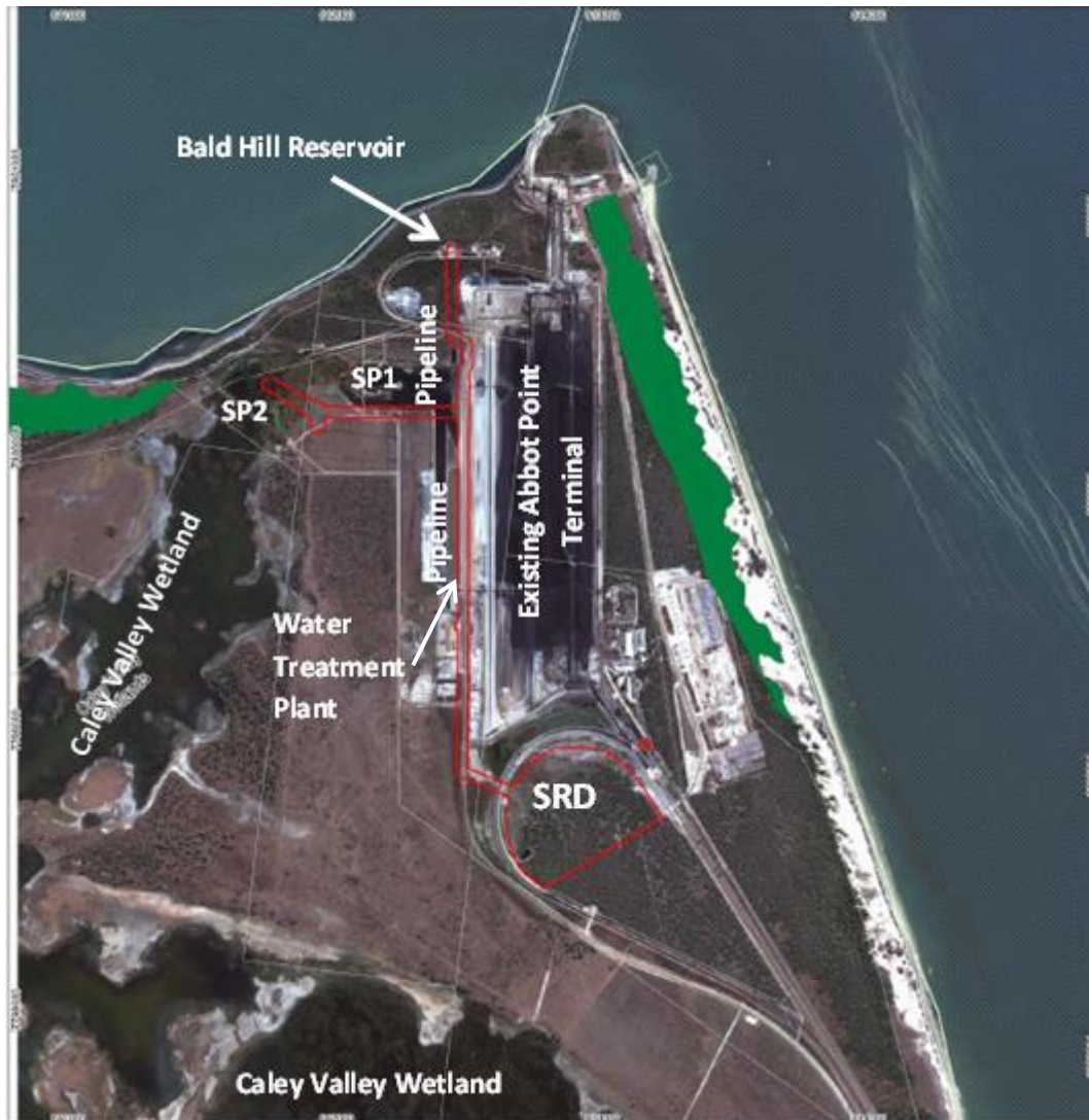
Figure 1 – Abbot Point Stormwater Return Dam
