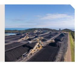
When it is ready for loading, coal is moved from the stockpile to a large surge bin. From here it is carried by conveyor along the 2.75 kilometre trestle jetty to the wharf and one of the two berths. Berth 1 is 252 metres in length and Berth 2 is 268 metres.
