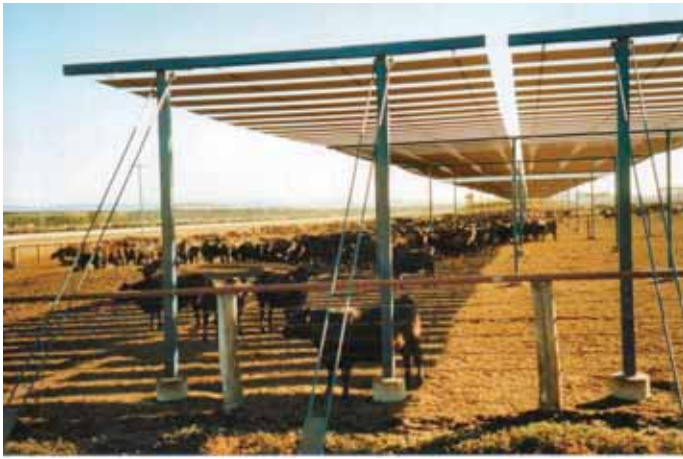
Figure 2: Feedlot iron sheet shade structure Photo courtesy of Sandalwood Feedlot, Dalby, Queensland
