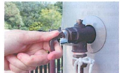
You will need to repeat this for a couple of days to ensure the tank fills to the top with water to enable the unit to operate correctly.
