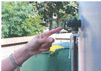
When you have located the **PRESSURE RELIEF VALVE**, you will need to grip the small handle and pull it firmly up to release the pressure inside the **HOT WATER UNIT (photo on the right)**, there will be an outlet pipe from the **HOT WATER UNIT** to the ground, please watch this pipe, steam and then water will flow from this pipe, when this happens, keep pulling handle until water flows freely from the pipe, this will allow the unit to fill with water.
