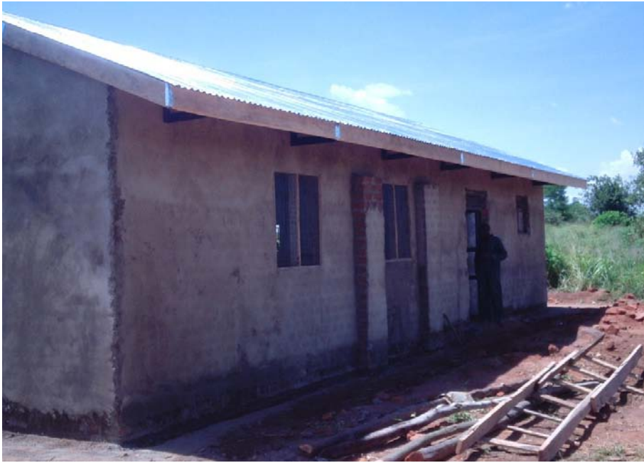
Above: classroom block under construction at the ECD Center.
