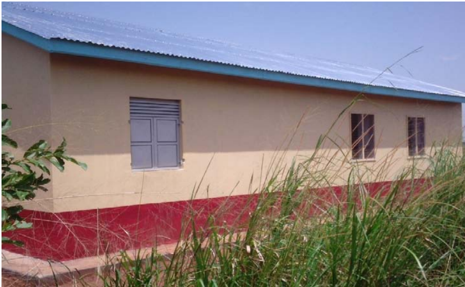
Above: Back view of the completed class room block
