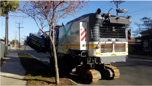
Some of the equipment used in the road repair work
