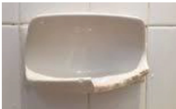
This broken soap dish in the shower could cause injury and needs to be replaced.
