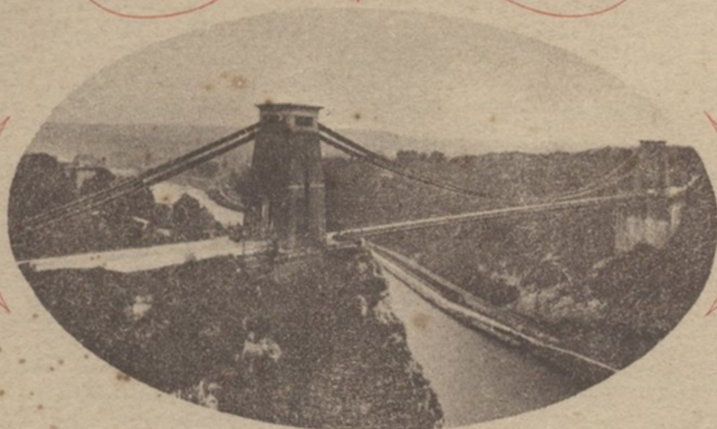
CLIFTON SUSPENSION BRIDGE.
