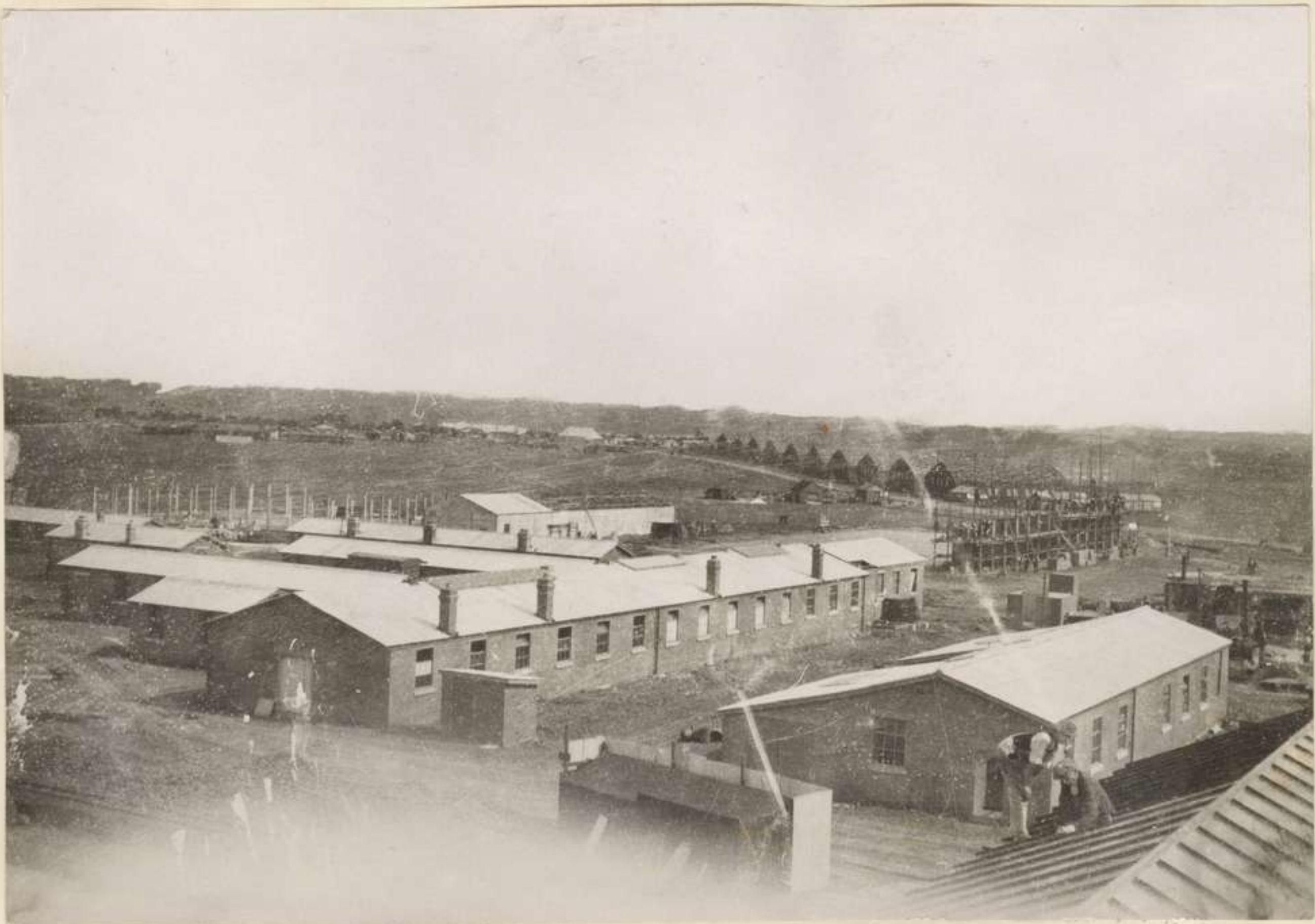
Mechin Haupton Station. Some of the Technical buildings. Instructional Huts & Offices in foreground.
