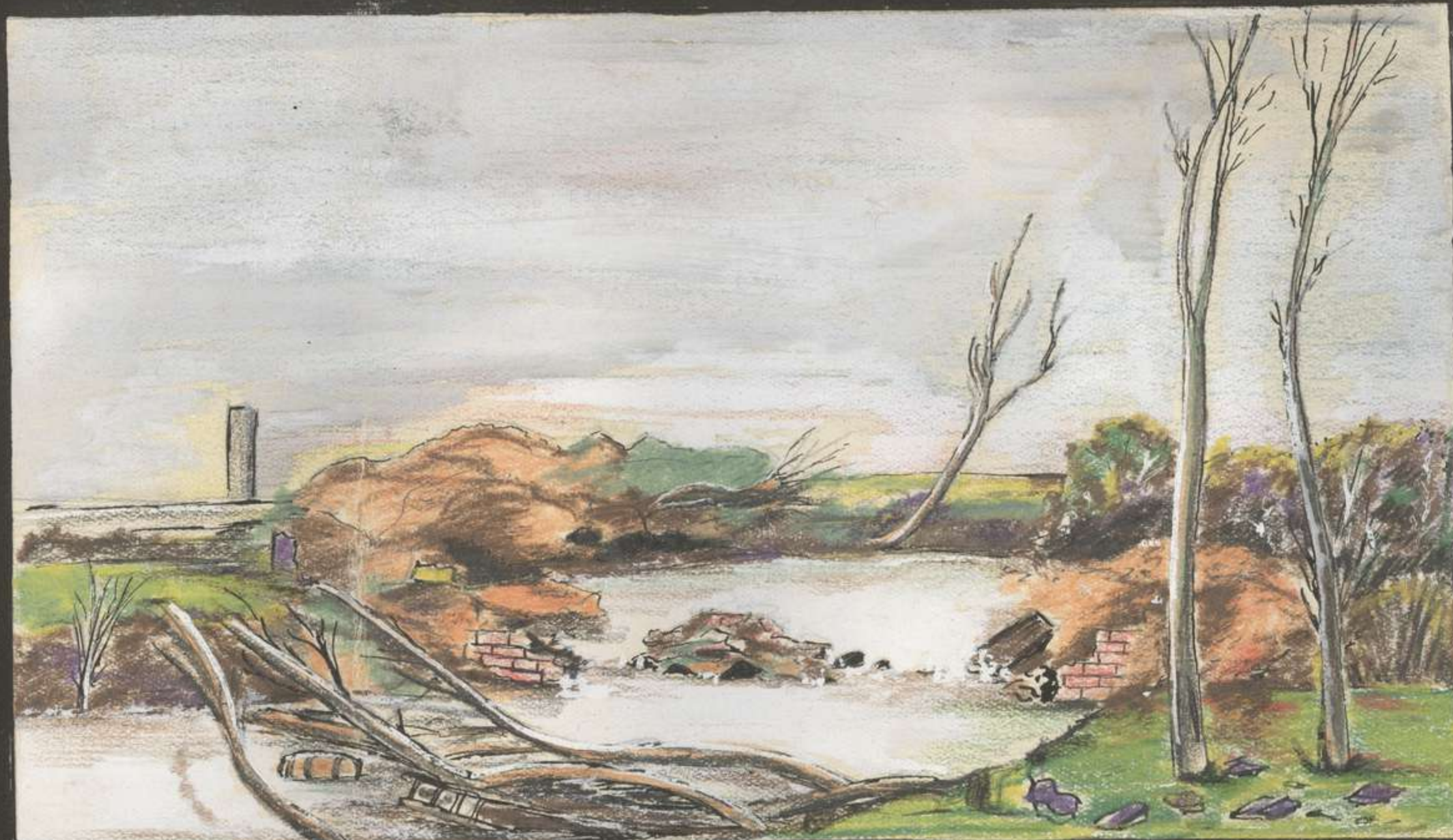
"THE BRIDGE OF PETIT FAYT BLOWN UP BY A MINE."
