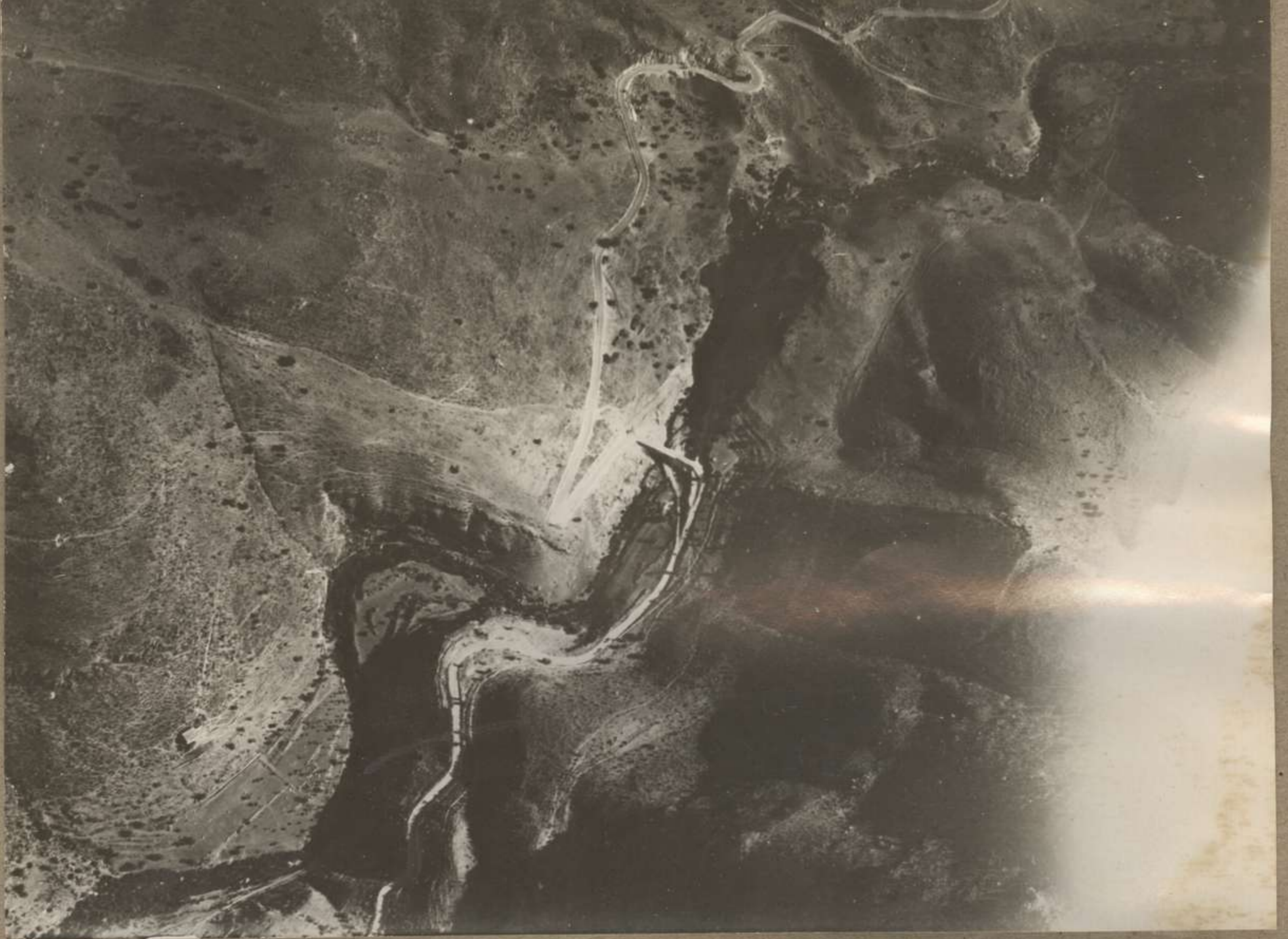
AINN 3196.07.30 h .11.9.18. BRIDGE. AT EL HOWEIJ, 9000 FT. FROM S.
