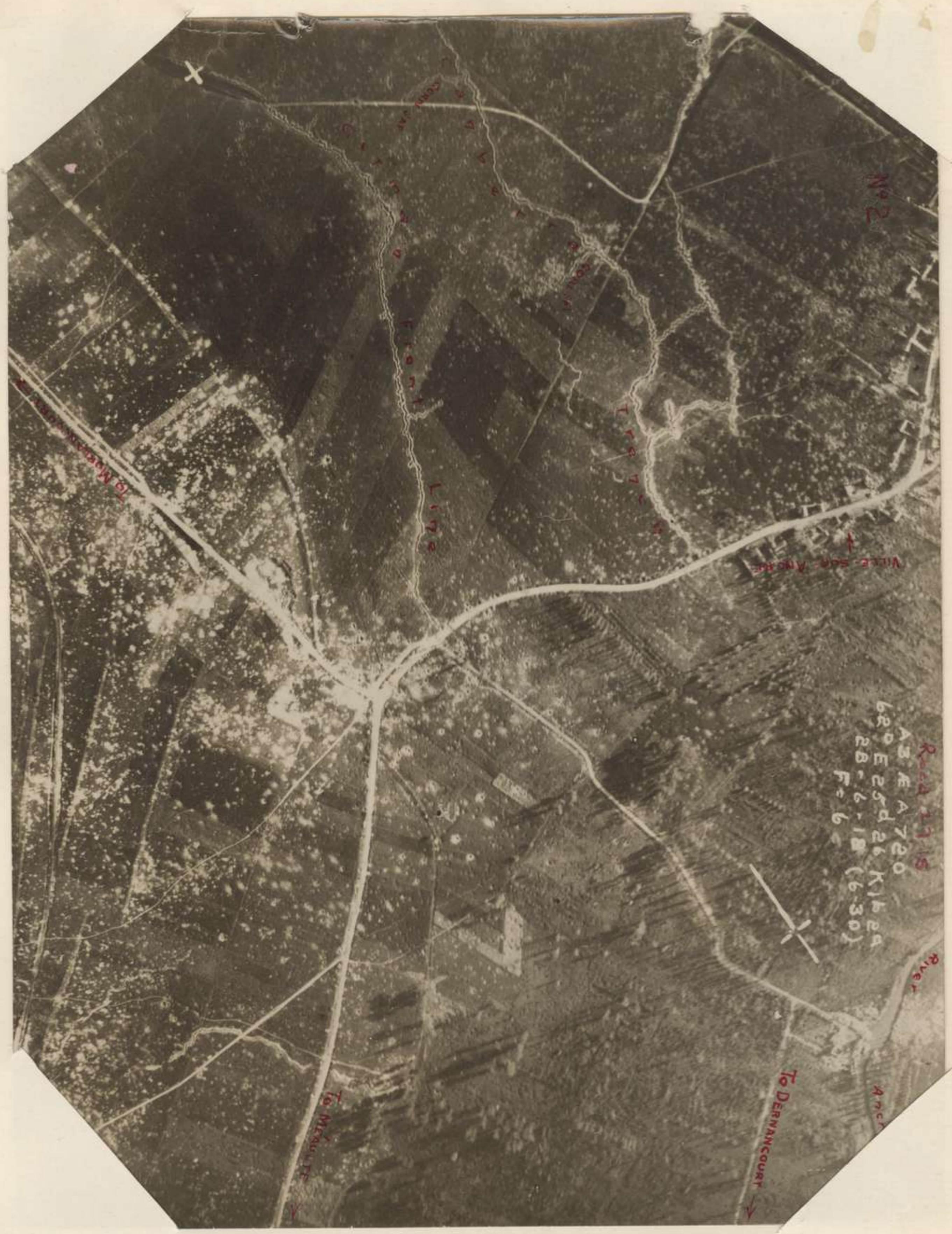
No.2 Shews CORN SAP excavated out as far as the road at which point a "T" head was put in to give the enemy the impression that it was merely a listening post. This "T" head can be seen in Photo 3. COAL SAP can also be seen in this photo excavated for about 70 yards out. A post to which COAL SAP was afterwards connected also shews up in this photo the post being put in mainly as a "blind". It will be noticed in this photo that the enemy had also commenced to sap forward more or less opposite CORN & COAL SAPS .
