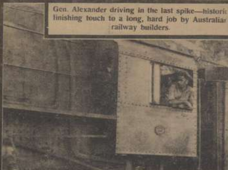
First engine to travel over the new stretch of line was driven by Gen. Alexander. Australian driver at window.
