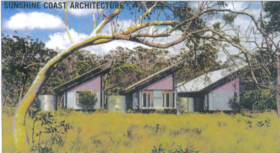
Lake Weyba design (left); the Hinterland House (below right); and Lake Weyba. Photos Courtesy Bark Architects and Reiner Blunk
