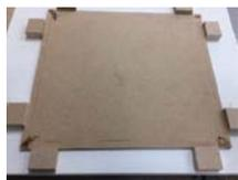
Create a template that is fractionally smaller than the internal dimensions of the AXIX™ sink.
