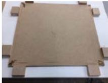
Create a template that is fractionally smaller than the internal dimensions of the AXIX™ sink.
