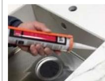
Apply silicone to the side joins of the sink and base joins where the steel sink meets the material.
