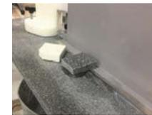
Using Corian® blocks, secure the AXIX™ sink to the worktop bonding with Corian® joint adhesive. Before bonding, ensure the areas are cleaned with IDA.
