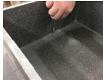
Using the inside of the box as a template, mark your cut out allowing a 2-3mm overhang.
