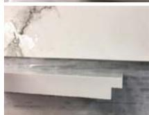
Rebate each end of the panel from top to bottom to accommodate the remaining two panels.
