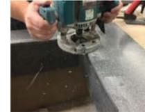
Worktop facing upwards, use router to trim excess overhang to a flush finish.
