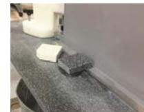
Using Corian® blocks, secure the AXIX™ sink to the worktop bonding with Corian® joint adhesive. Install the rubber gasket under the block where it secures to the sink. Before bonding, ensure the areas are cleaned with IDA.
