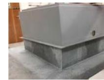
Turn worktop upside down, sleeve the AXIX™ sink over the box to check for size. Remove AXIX™ sink.
