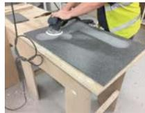
Sand the worktop around the area where the box will be bonded which will remove any imperfections.
