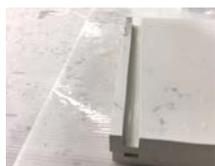
Cut two adjacent panels to the correct length and depth.
