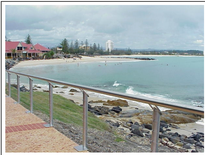
Stainless Steel Wire Balustrade with Stainless Steel Handrail:
