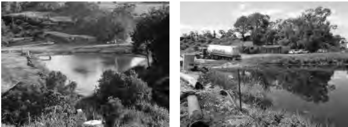
Photo 1 Leachate pond and excess leachate is taken away during high rainfall period
