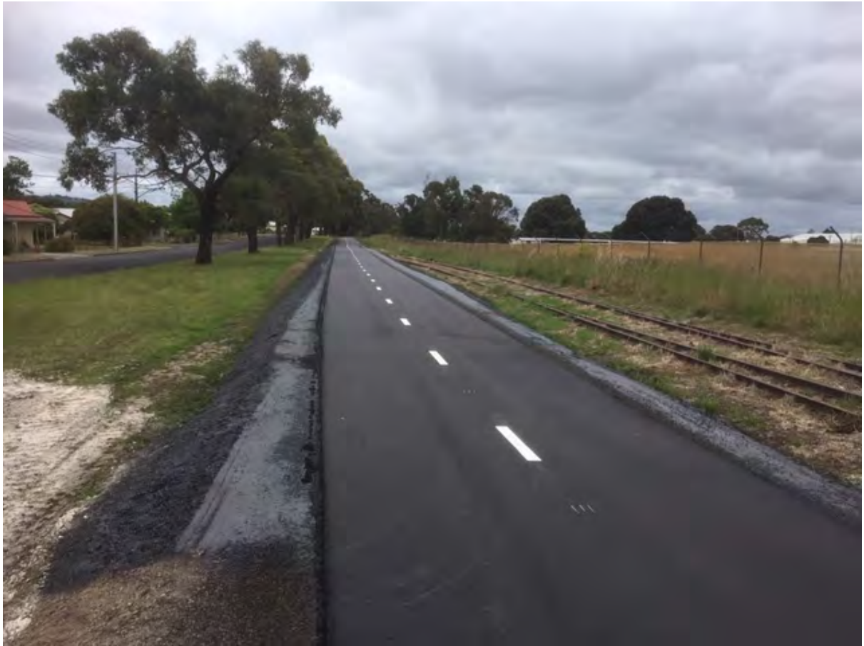
Figure 2: Rail Trail looking West to Pick Ave
