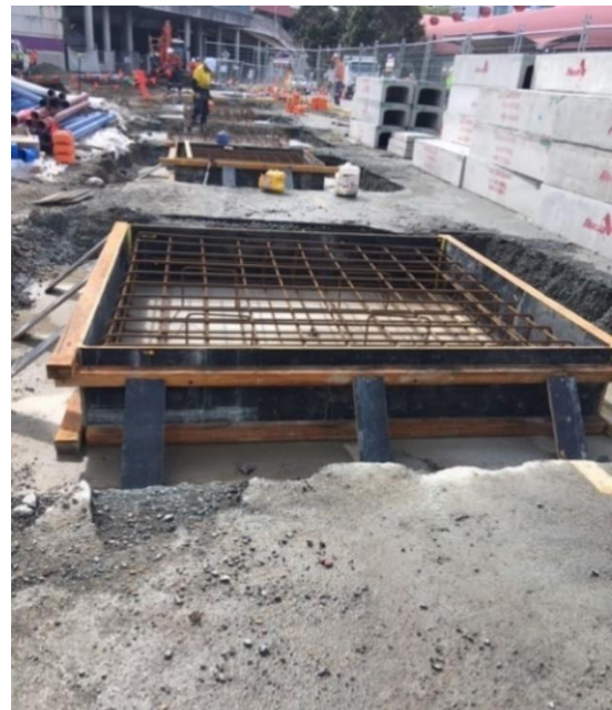
Figure 3 – Pad footing preparation
