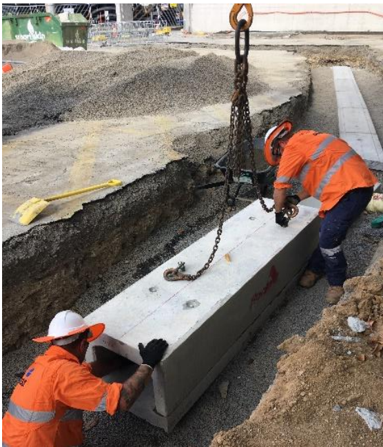
Figure 2 – Stormwater drainage installation
