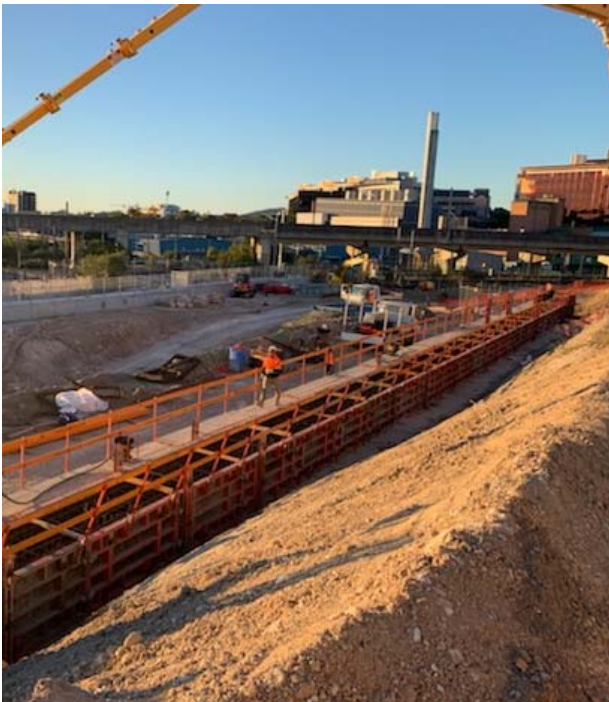
Image: Installing the pile capping beam
