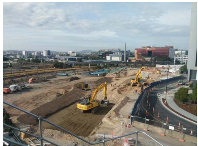
Image: Work underway at the Boggo Road station site
