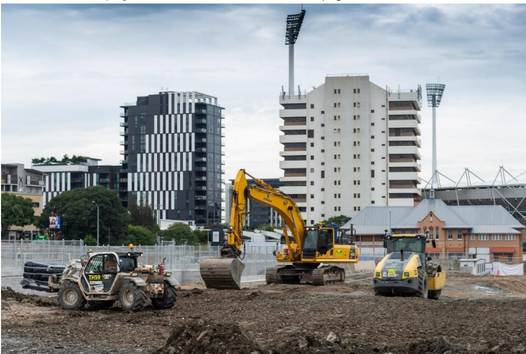
Image 1 Construction equipment undertaking surface works at the Woolloongabba site
