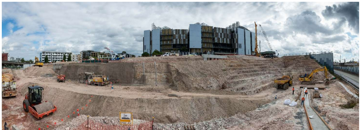
Image above showing work underway at the Boggo Road station site
