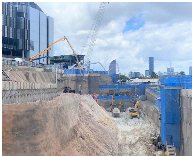
Image: Work continues at the Boggo Road station site
