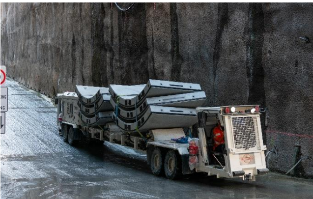
Image 5 Tunnel segments being delivered to the TBM
