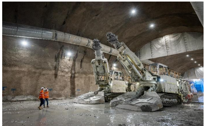
Image 6 Two roadheaders currently tunnelling south to Boggo Road
