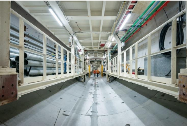
Image 1 TBM 1 Else - inside the TBM
