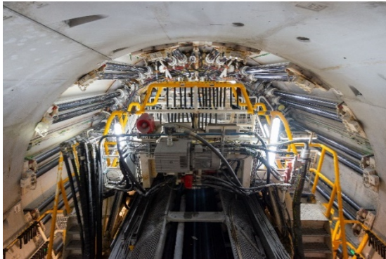
View from inside the front of TBM 1 Else
