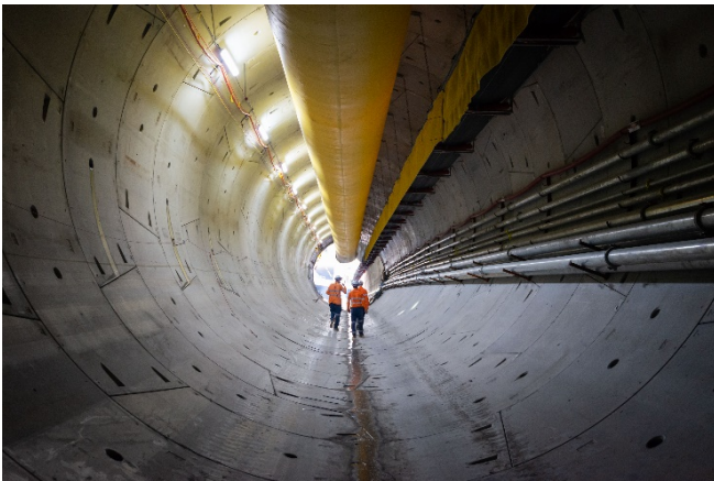
TBM tunnelling works are well underway
