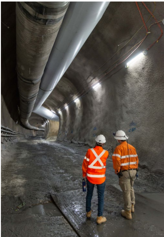
Underground tunnel view from Woolloongabba towards the new Boggo Road station
