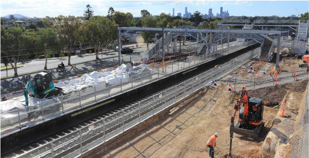
Image – Completed demolition of station buildings and piling being undertaken at Yeronga during June 2021
