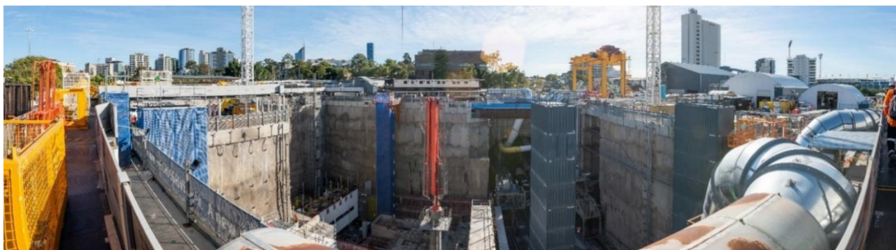
Image 2 Panoramic view of the Woolloongabba station box building site
