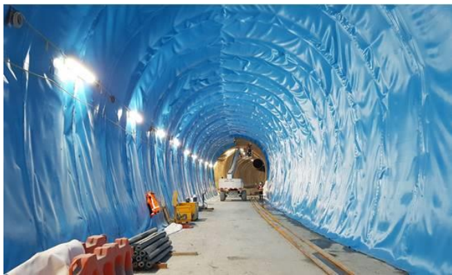
Image 1 Waterproofing underway in the mined tunnels
