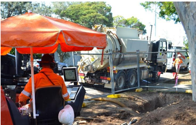
Services under bore drilling works on Ashby Street
