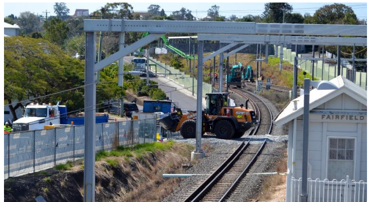
Overhead electrical line mast foundation works in the rail corridor
