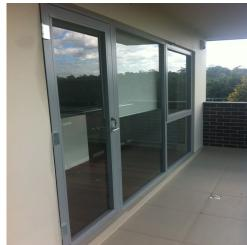
The Warrior range of bushfire doors is fully approved for fire ratings of -/30/- and has been full scale fire tested in strict accordance to AS1530.4.
