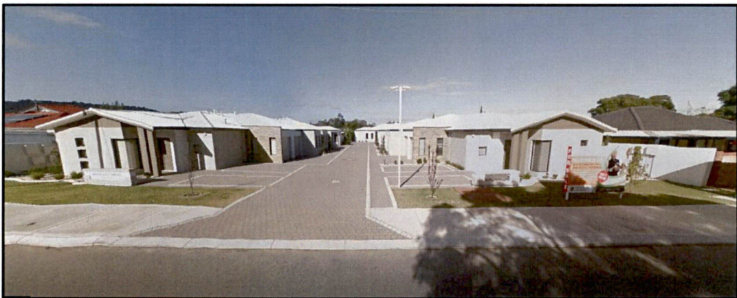
Figure 3: View of the Subject Site from Maida Vale Road
