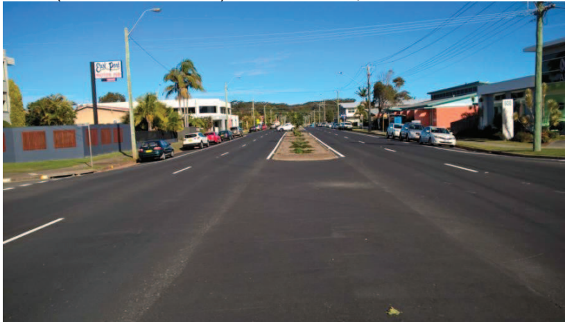
Pavement Rehabilitation, Lord St, Port Macquarie
