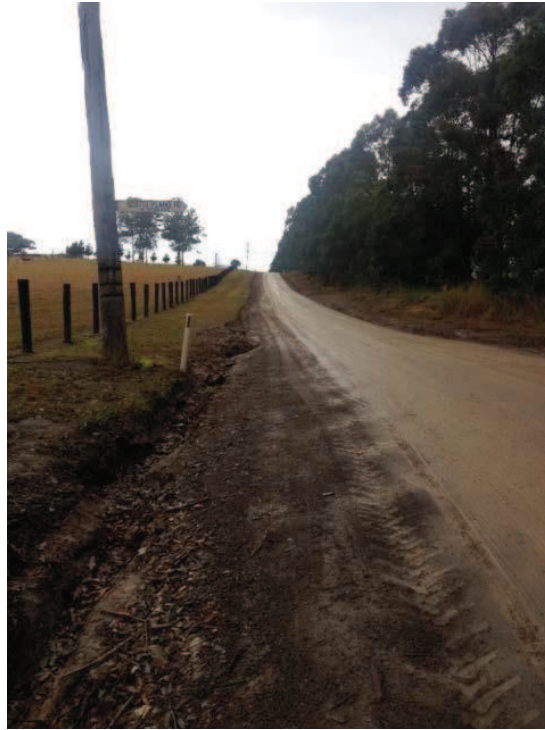
Gravel Resheet, Ballengarra Bransdon Road, Telegraph Point
