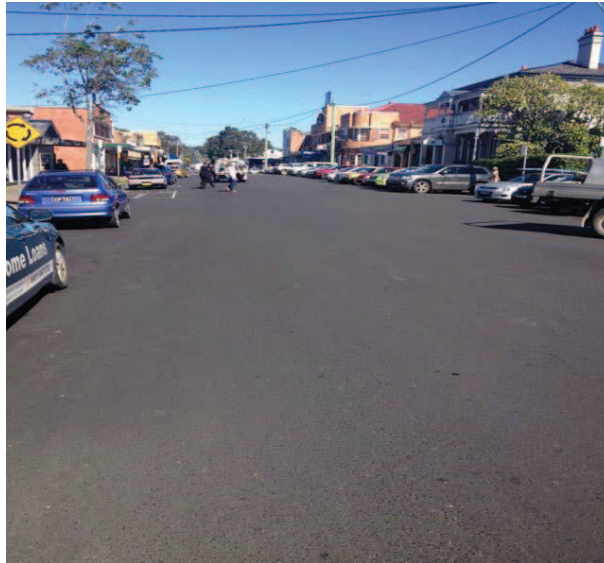
New Asphalt, Cameron Street, Wauchope
