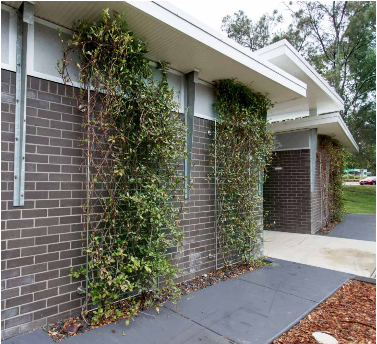
Integrated rain gardens at Warners Bay amenities buildings (constructed in 2013)
