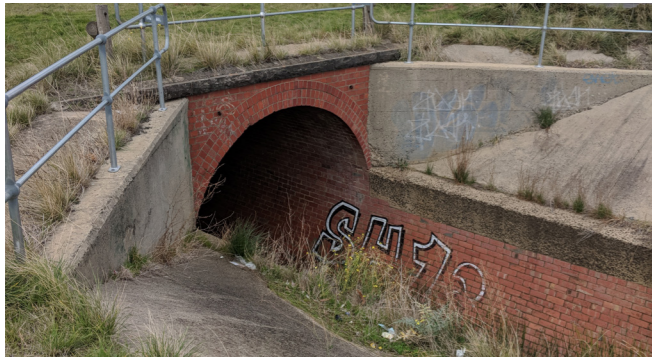
EXISTING BRICK LINED BRIDGE
