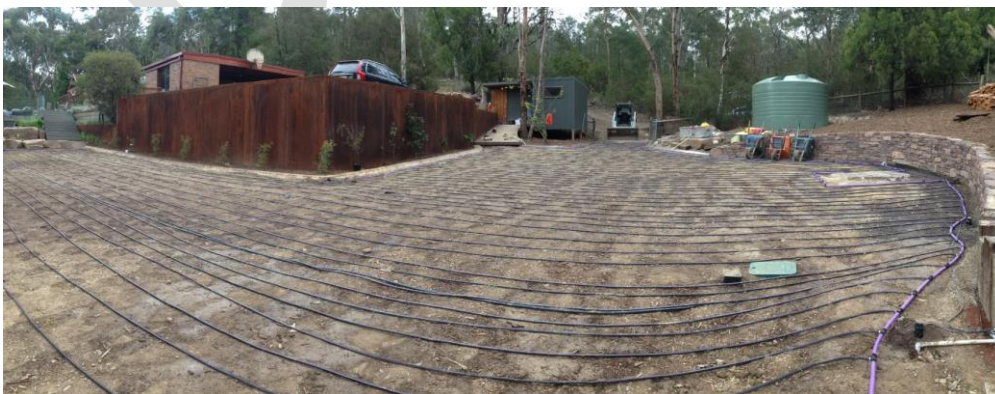
Figure 4: Lay-down of sub-surface irrigation
