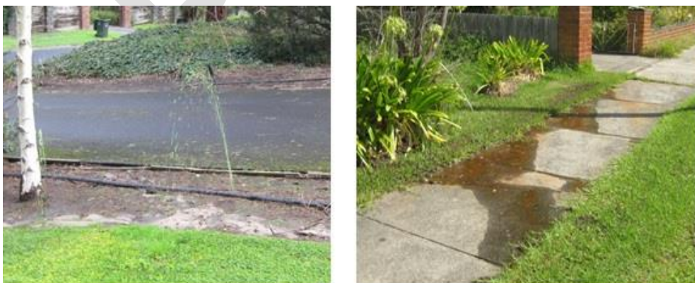
Figure 6: Burst dripper line and septic effluent flowing over footpath
