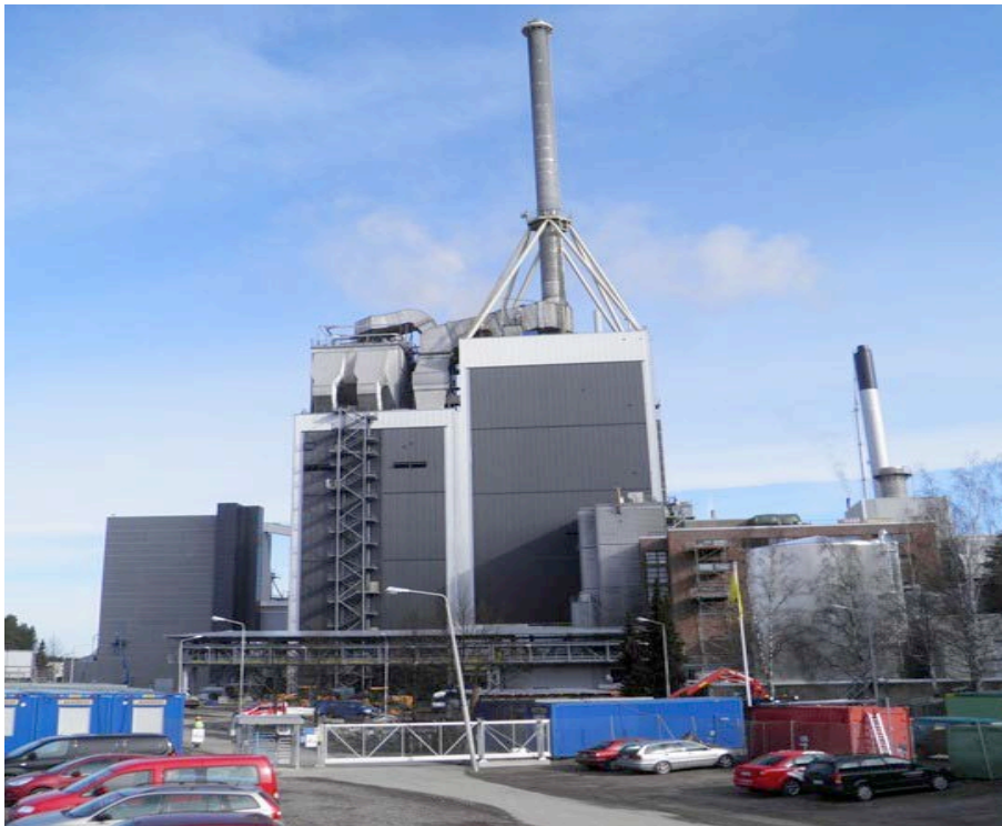
FIGURE 77: KYLMÄJÄRVI 2 MUNICIPAL WASTE GASIFICATION RENEWABLE GAS FUELLED COGENERATION NETWORK, LAHTI, FINLAND (SOURCE: LAHTI ENERGIA)
