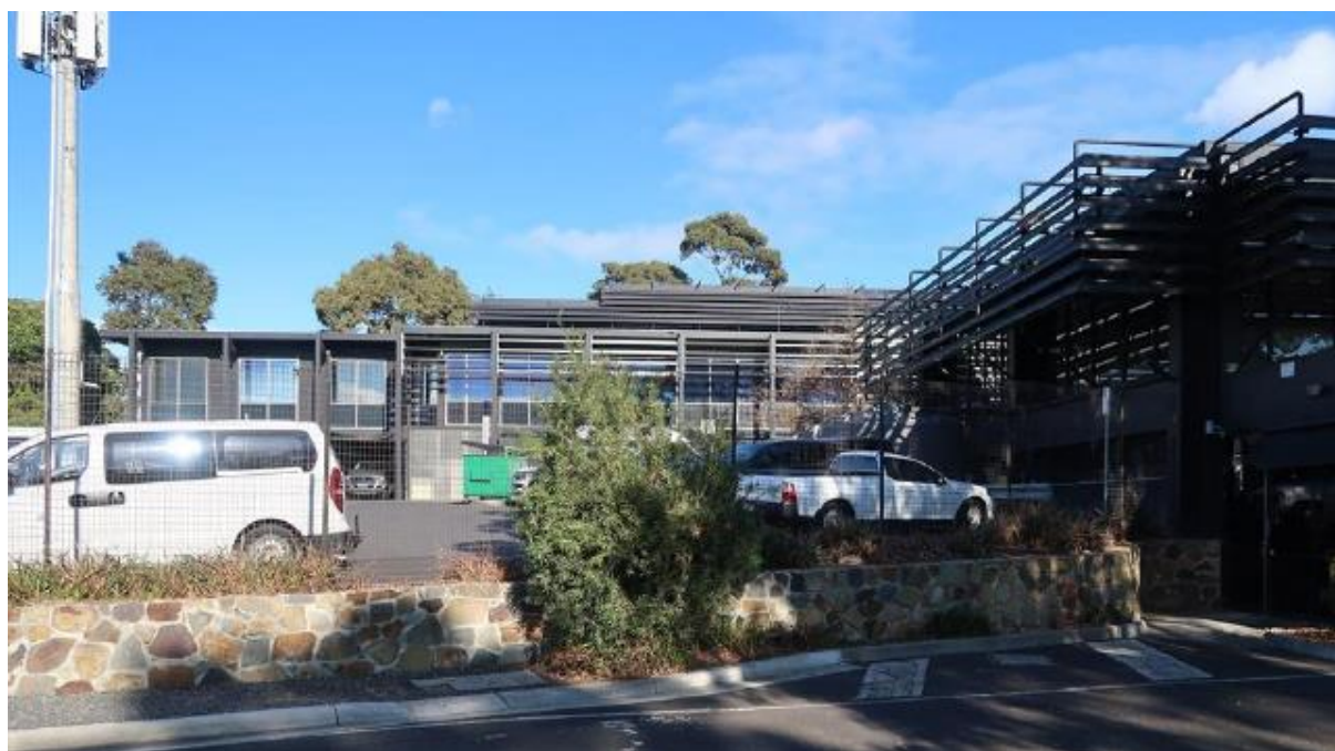
Figure 4 View of the rear (north elevation) of the Council offices showing remnants of the 1964 addition to the left and the 1977 additions to the right and the use of louvres.
