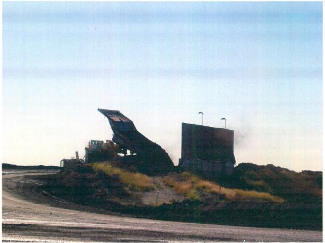
Photograph D.3 View of ROM bin in operation at WML
