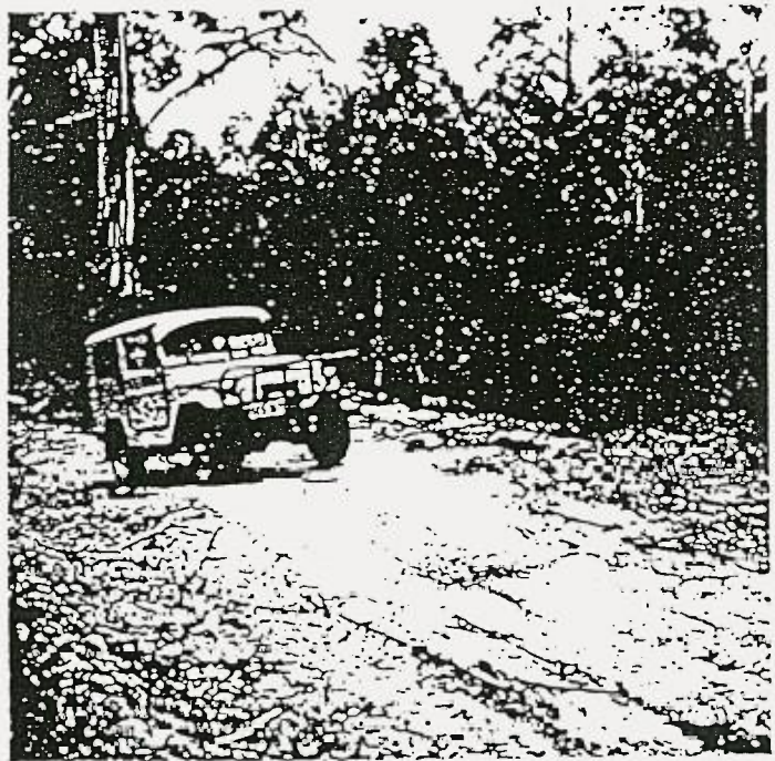
Figure 6 Trafficable cross banks can be comfortably negotiated and provide effective drainage when sited and built correctly.
