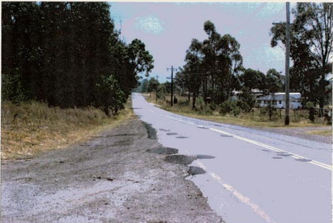
Photo 7: View of Greendale Road west from the plant entrance.
