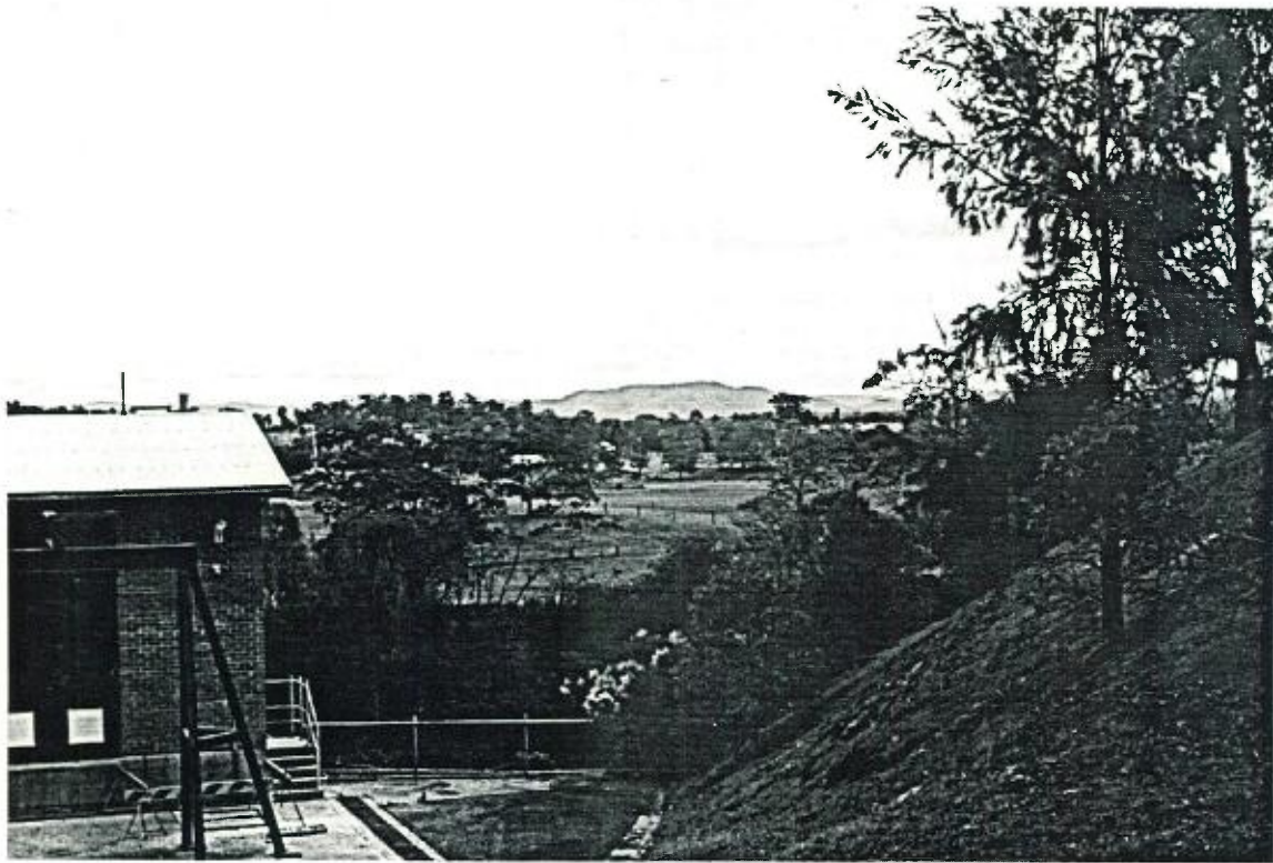
a. Views from the existing pumping station of residences on Koree Island
