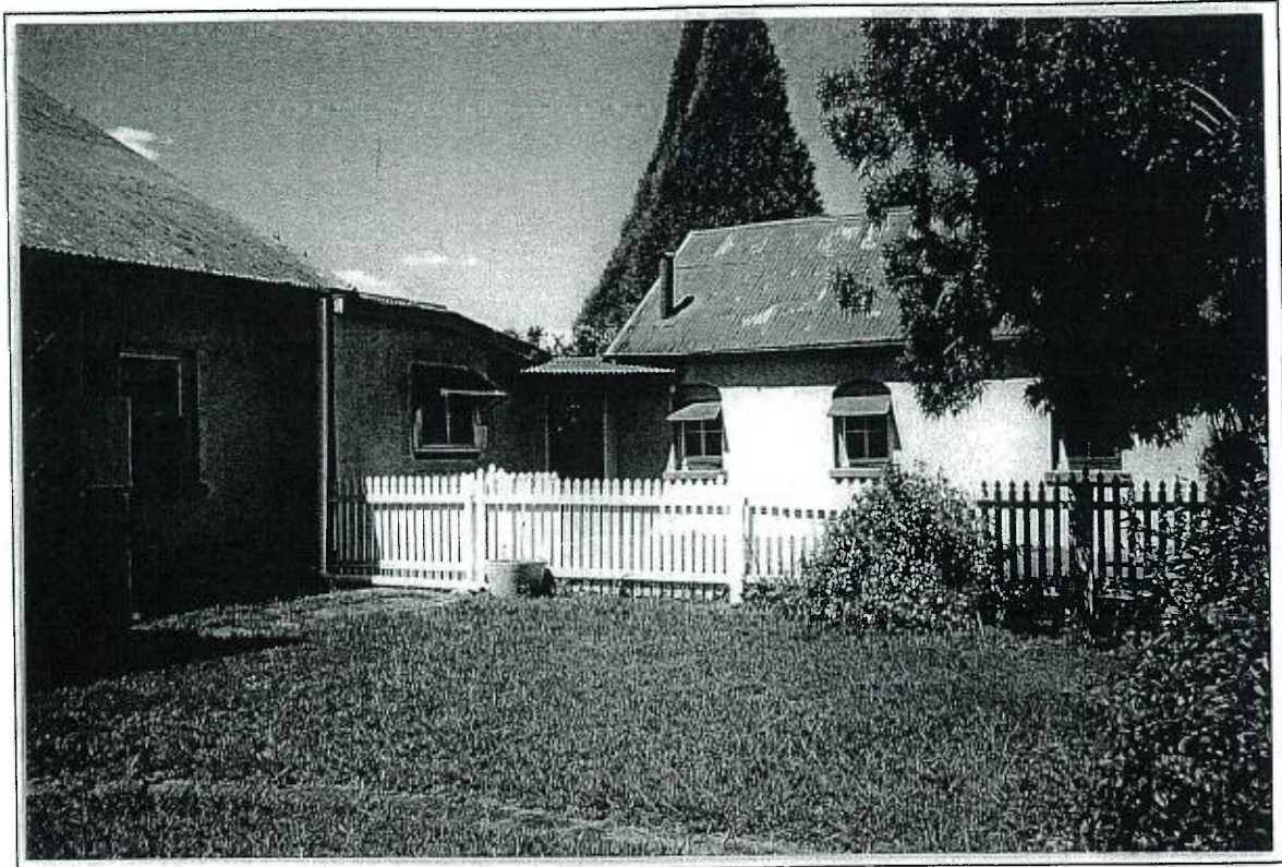
Fig 4.5 View of later kitchen link to early kitchen wing looking east
