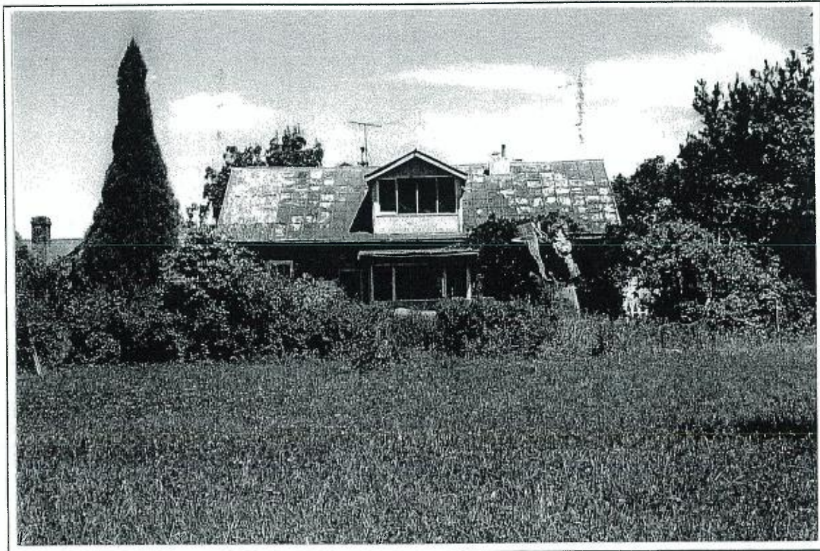
Fig 4.1 View of north elevation of Vine Lodge with original roof form and verandah removed, new enclosed balcony and extension to east where the former kitchen was located
