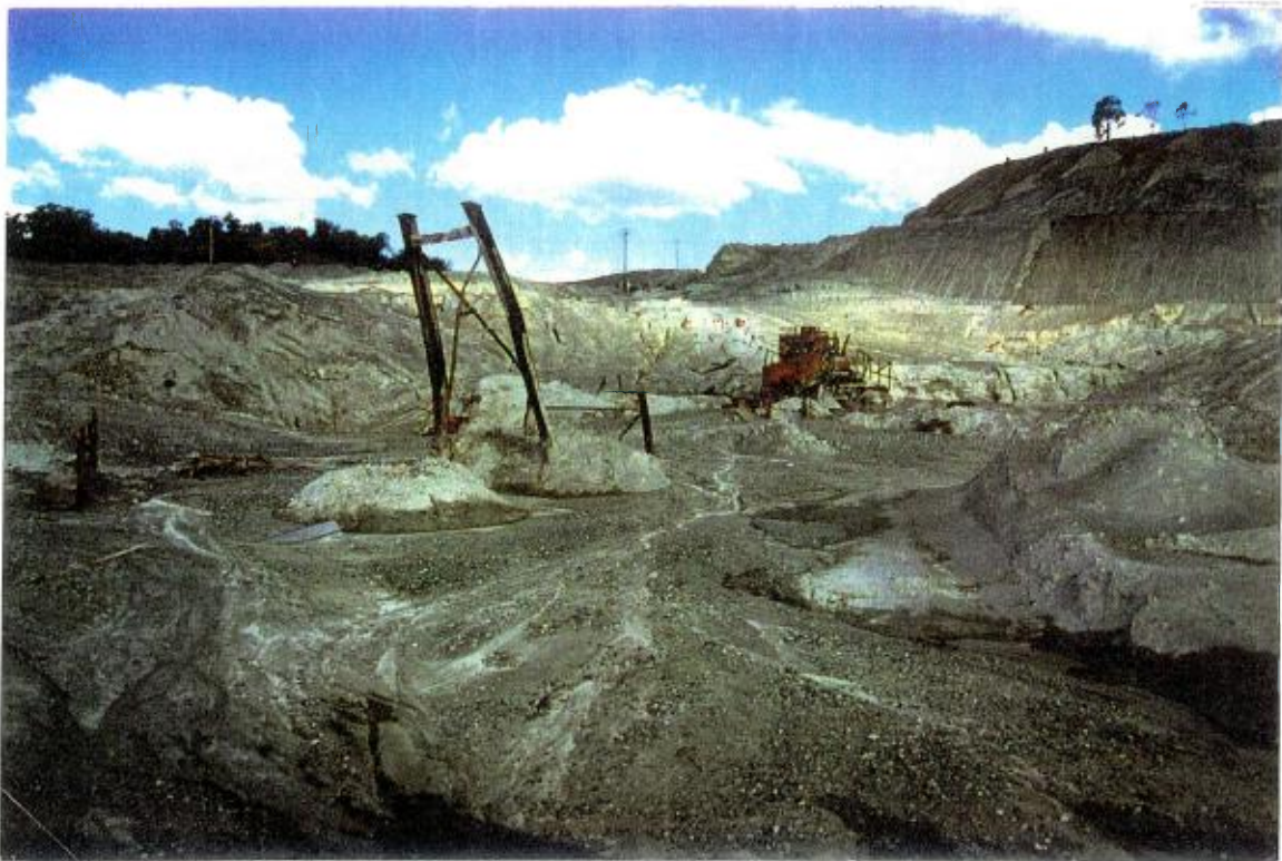
Figure 4.5: Erosion of the access track and conveyer belt run, at the north west end of the tailings dump.
