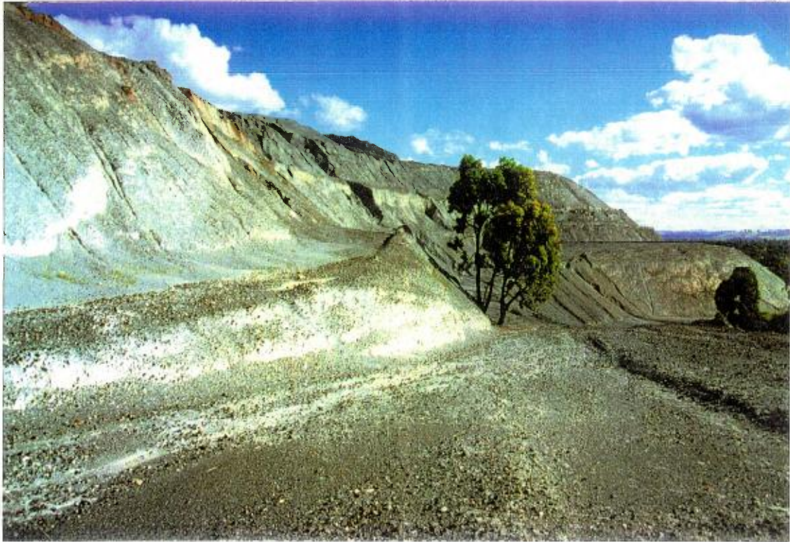
Figure 4.4: Rill erosion along the western batters of the tailings dump.
