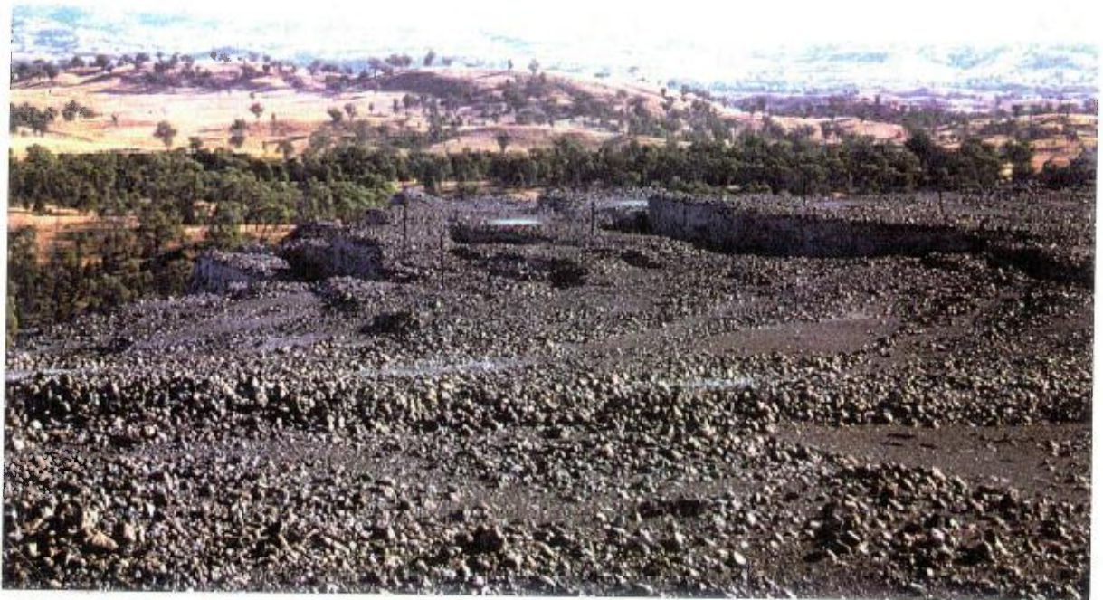
Figure 4.7: Steel gauge posts on the southern batters of the tailings dump.
