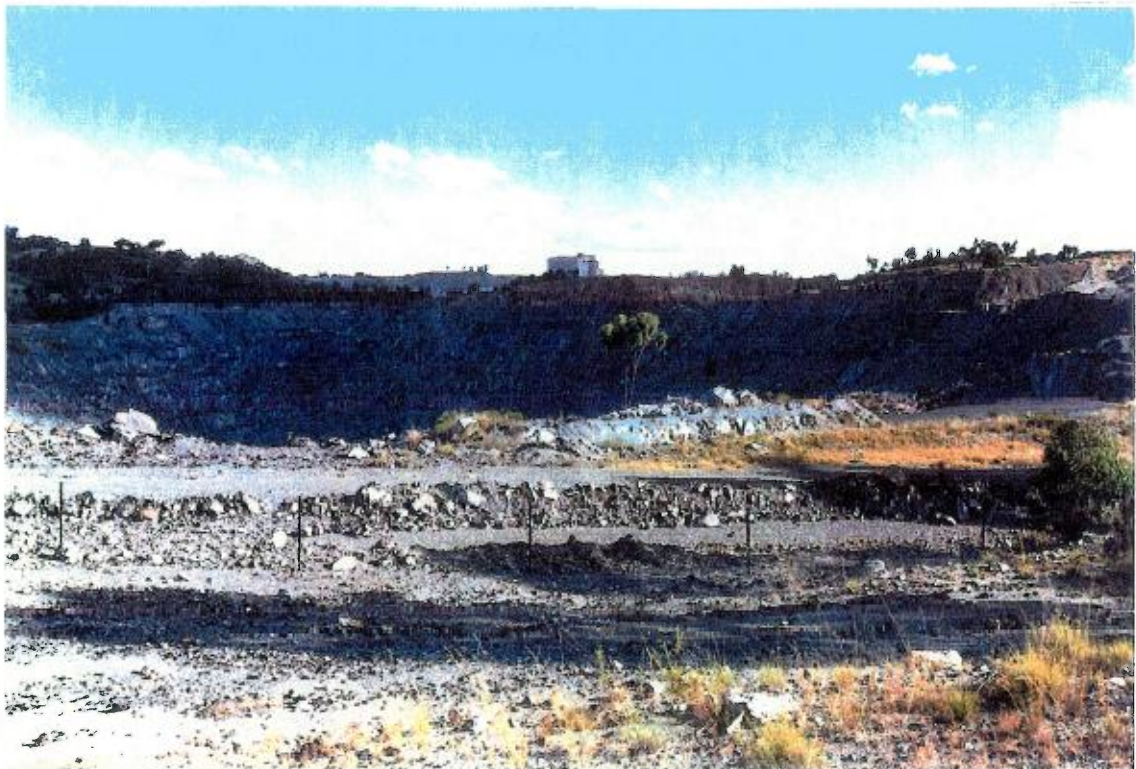
Figure 7.2: Plain wire perimeter fencing above the North Pit
