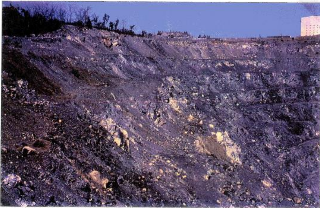
Figure 5.4: Mass movement within the North Pit
