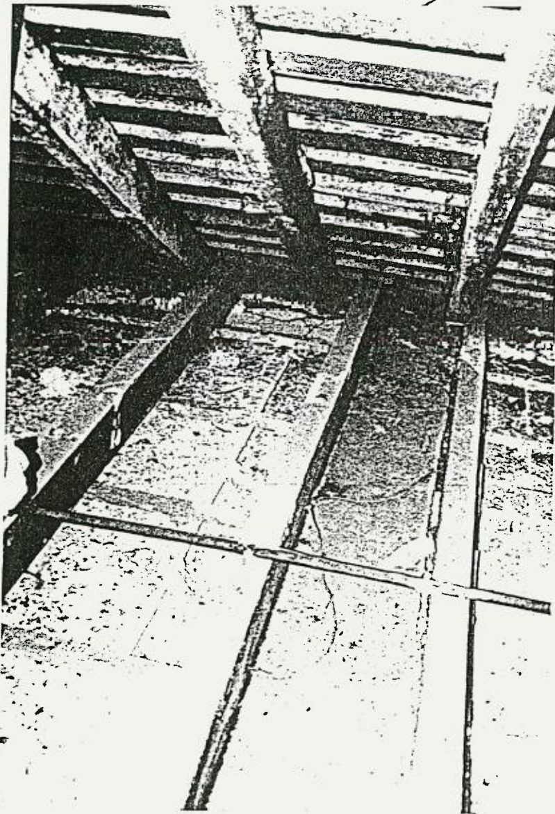
Photo 14, Roof space, "Minnaville" homestead. Double brick wall between Phase 2 & Phase 3 construction
