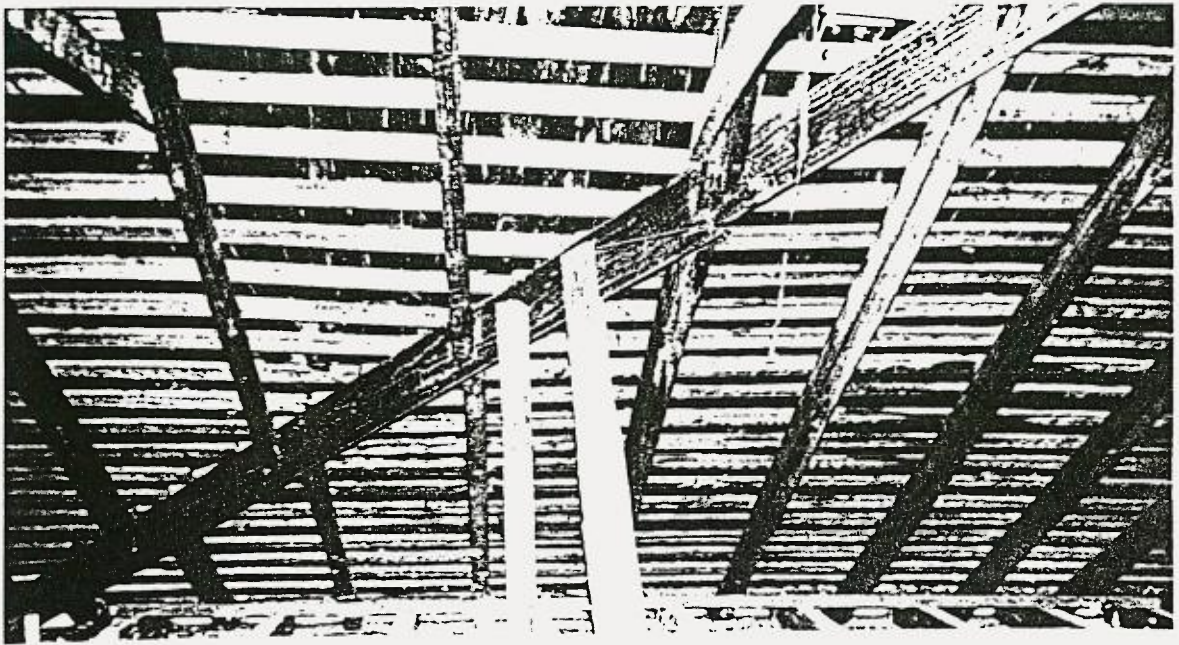
Photo 11, Roof space, "Minnaville" Phase 1 cottage, showing hipped rafter (on diagonal).
