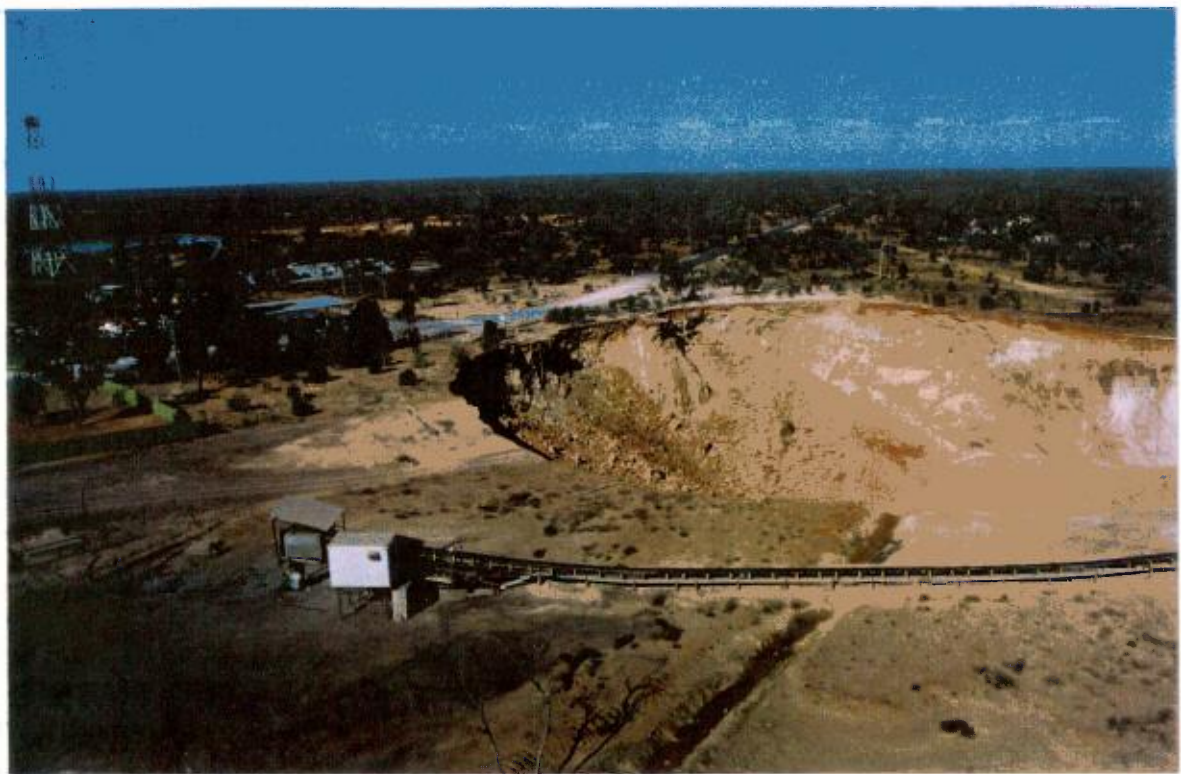
18 March 1996 Subsidence looking West from Cement Silo
