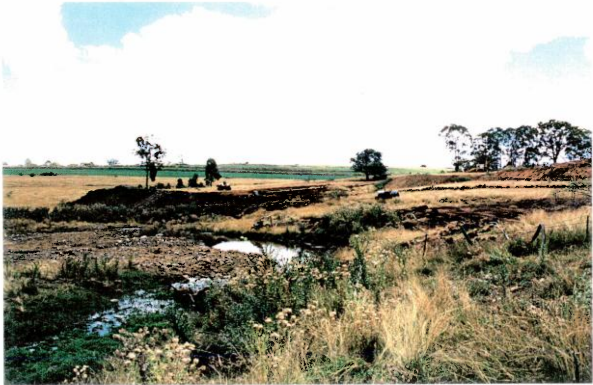
5. SPRING GULLY & DAMS UNDER CONSTRUCTION
