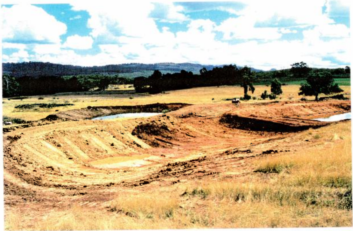
3. DAMS UNDER CONSTRUCTION
