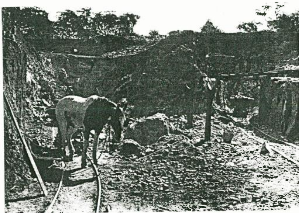
Figure 3.5: Torrington Wolfram Pty. Ltd. Number 2 quarry, ML 75, 1910. Note the V-shaped skips, one of which is being pushed by hand, and another which appears horse drawn.
