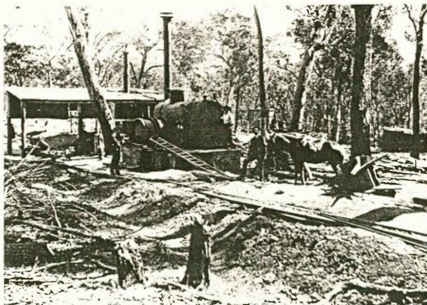
Figure 3.6: Rockvale Wolfram Company's hauling plant, Carter's section, 1910. Note the winding drums attached to the Robey winding engine.
