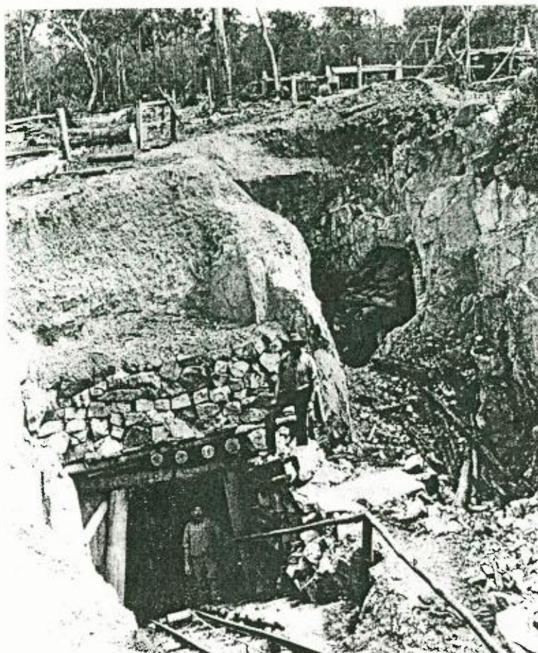
Figure 3.3: The incline (underlay) shaft at the Torrington Ore Company's Bismuth Mine, 1910
