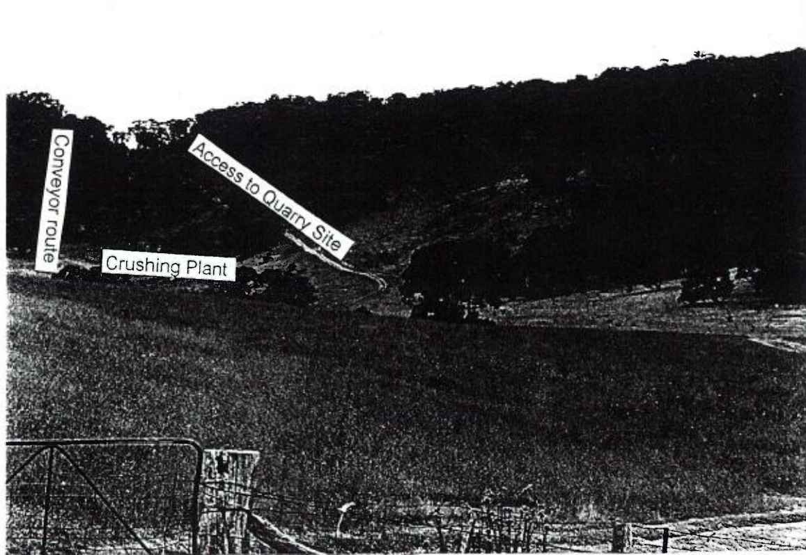
Photo 7: Site of crushing plant and conveyor
