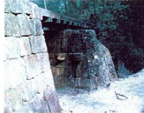
Clares Bridge (Precinct 3.7.0)
