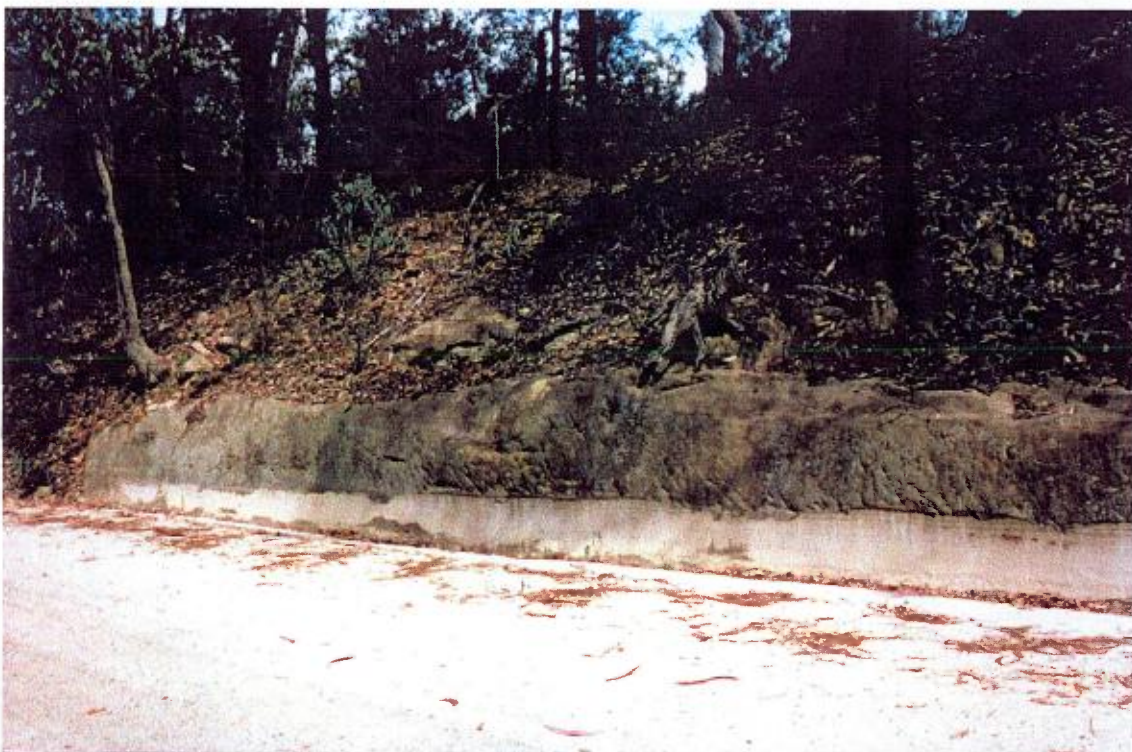
Pick-marks above grader blade damage which has removed the face of the cutting.
