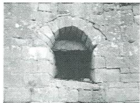
Arched Culvert, Murrays Run (Precinct 4.6.0)
