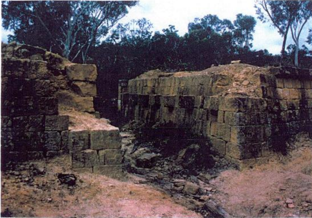
Circuit Flat Bridge (Section 3).
