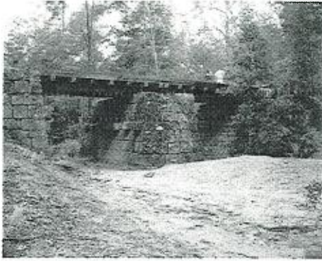
Clares Bridge (Precinct 3.7.0)
