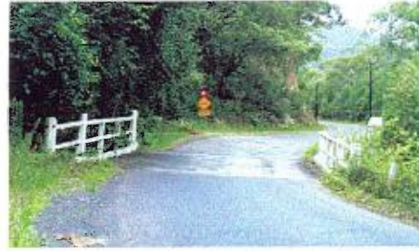
Settlers Road Bridge (Precinct 3.2.0)
