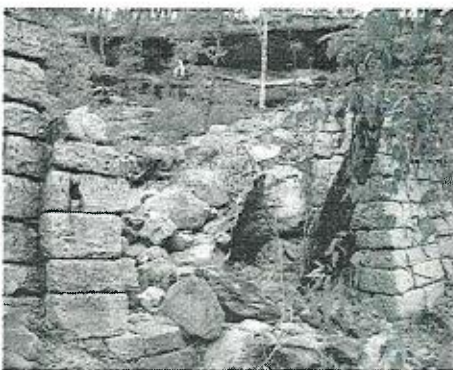
Sampsons Pass Bridge (Precinct 3.10.0)
