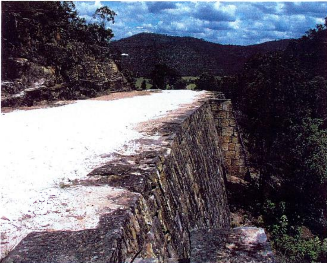
Devines Hill , near Wisemans Ferry, Dharug National Park Before and completion of recent remedial works, including removal of invasive vegetation, clearing of drains, and addition of new fill / wearing surface for road.
