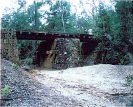
Clares Bridge (Precinct 3.7.0)
