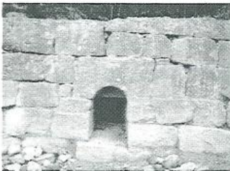
Arched Culvert, Fernances (Precinct 4.5.0)
