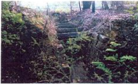
Old Northern Road Bridge (Precinct 1.3.0)
