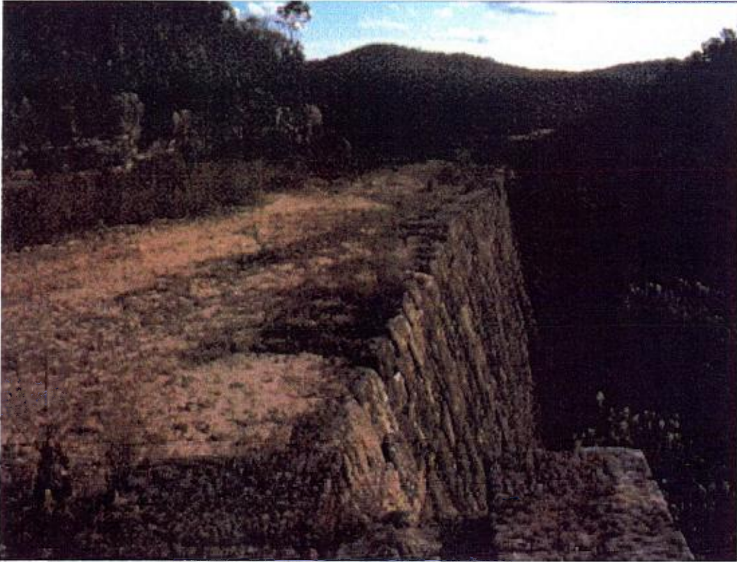
Devines Hill , near Wisemans Ferry, Dharug National Park Before and completion of recent remedial works, including removal of invasive vegetation, clearing of drains, and addition of new fill / wearing surface for road.
