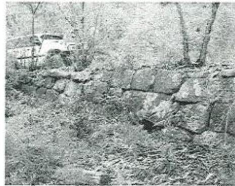
Wall & Culvert south of Sampsons Pass
