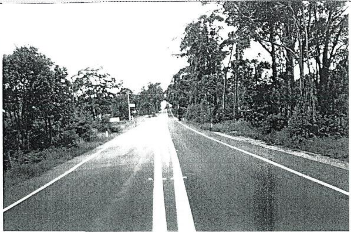
PHOTO P2 - View south along Old Northern Road from northern end of striped median about 130 metres north of Roberts Road. Opening in median at Roberts Road on left.
