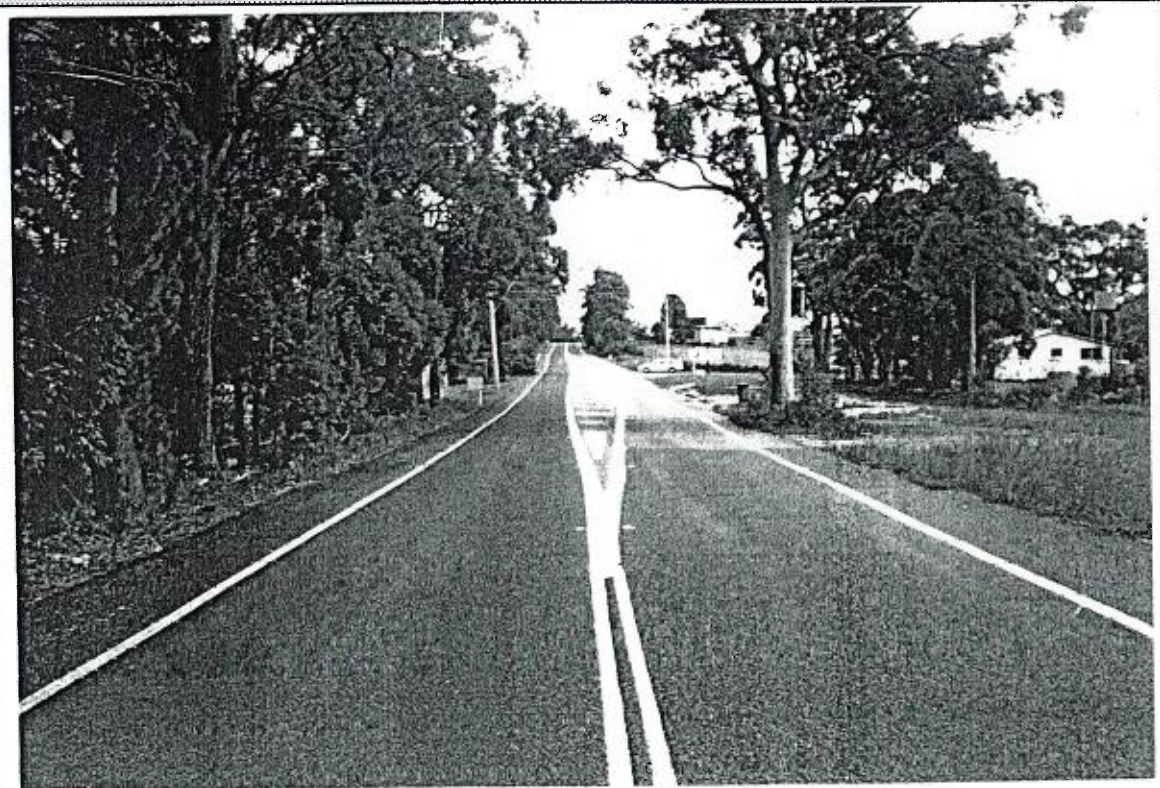
PHOTO P1 - View north along Old Northern Road from southern end of striped median. Opening in median at Roberts Road on right.
