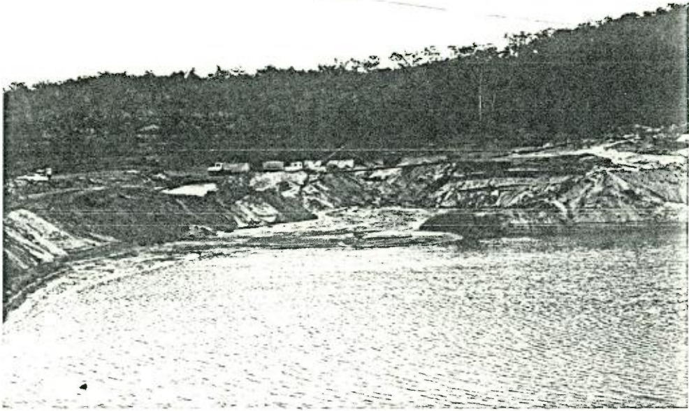
PLATE 7: Open pit of existing sand extraction operation, looking southeast.
