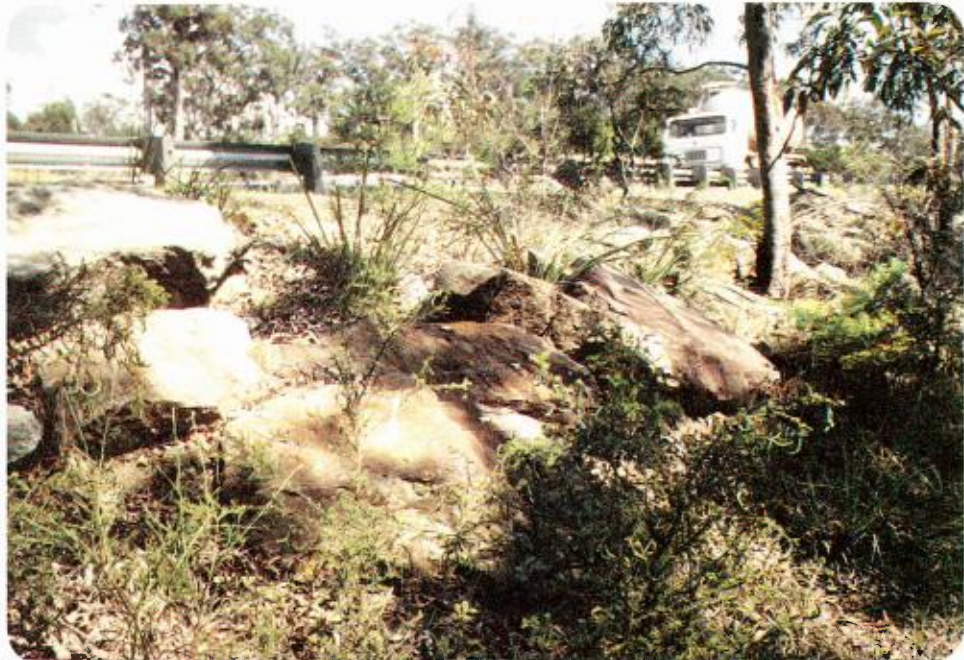
(14) Regeneration on sandstone batter (SECTION 9.2.8)
